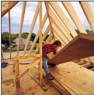
A new home under construction
